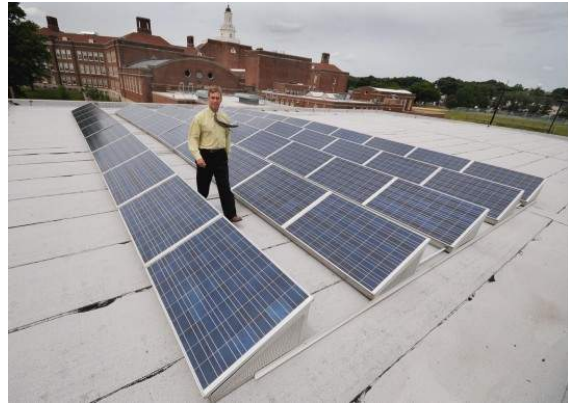
The News Journal/FRED COMEGYS John Read, construction project manager for Brandywine School District, walks among the solar panels on the roof of the newly renovated P.S. du Pont Elementary School. The district is considering them for Brandywood Elementary.
